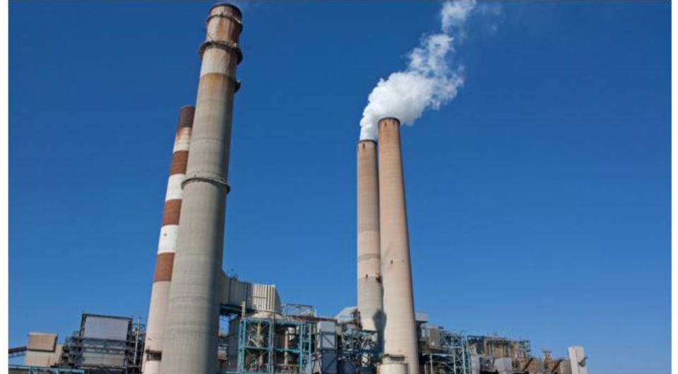
Big Bend Power Station is a major coal-fired power plant near Apollo Beach, Florida.
